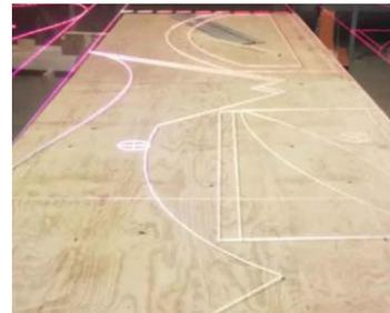
Figure 3: AR-Projection of free-form building parts onto LVL-boards
